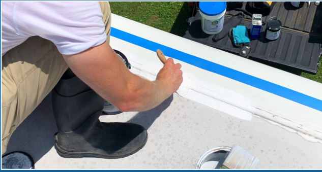
APPLY A THICK AMOUNT OF CRAZY PATCH OVER TERMINATION BARS
