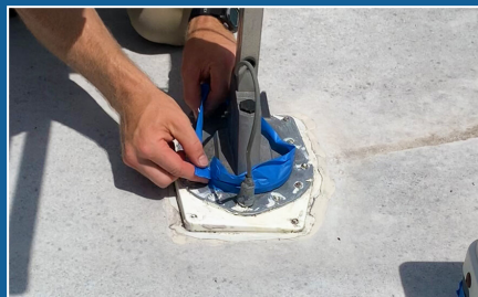
TAPE AROUND ANTENNAES
