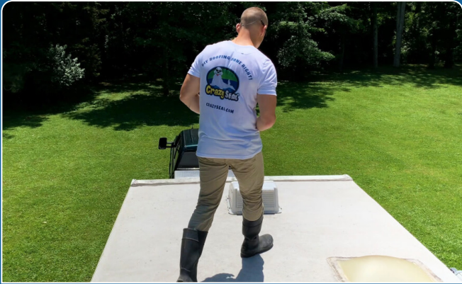
WALK THE ROOF & IDENTIFY ANY PROBLEM AREAS
