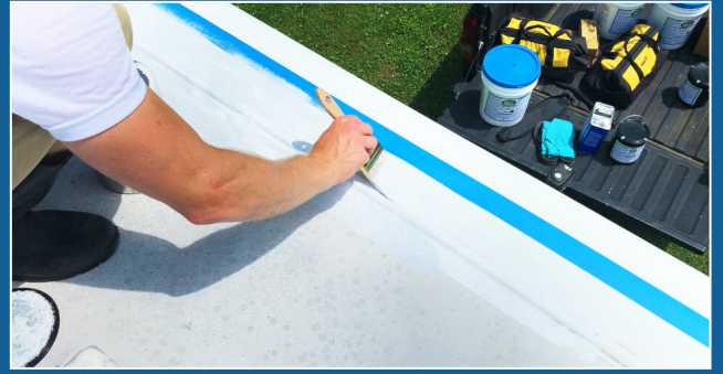
PAINT OVER CRAZY PATCH WITH CRAZY SEAL WHILE STILL WET
