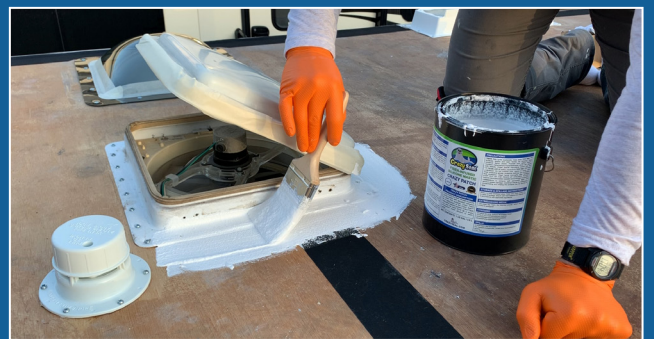
REPEAT WITH ALL FIXTURES ON THE ROOF WHERE PENETRATIONS ARE PRESENT
