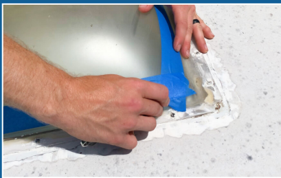
USE A KNIFE TO CUT ROUND CORNERS ON SKYLIGHTS
