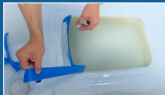
REMOVE TAPE WHILE STILL WET
