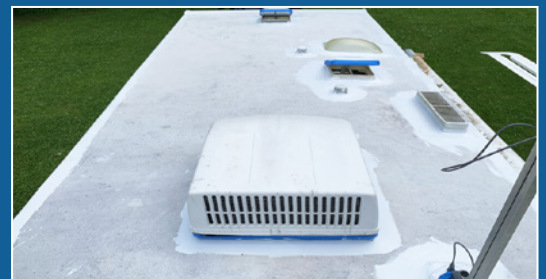
CUT IN ENTIRE ROOF TO PREPARE FOR CRAZY SEAL ROLL ON
