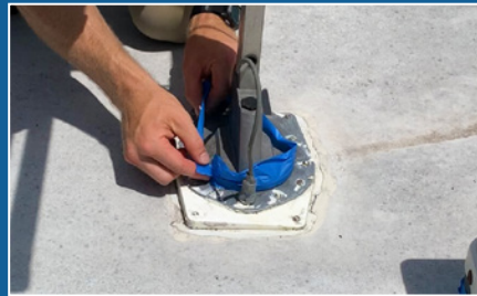
TAPE AROUND ANTENNAES
