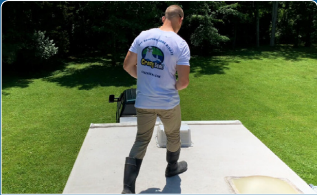
WALK THE ROOF & IDENTIFY ANY PROBLEM AREAS
