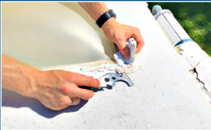
REMOVE LOW QUALITY SEALANT WITH PRYING MOTION & SCRAPER BLADE
