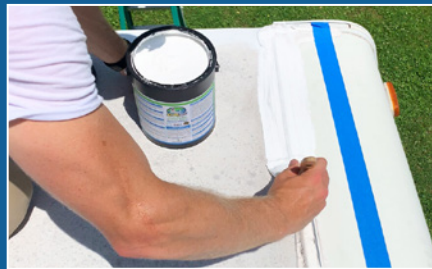
COVER ALL PENETRATIONS & TERMINATION BARS WITH CRAZY PATCH
