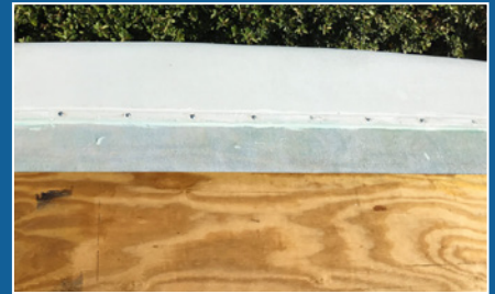
CRAZY TAPE APPLIED ON SEAM
