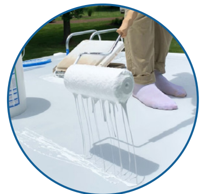
3. CRAZY SEAL SYSTEM INSTALLATION
