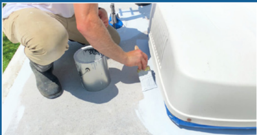
CUT IN AROUND FIXTURES
