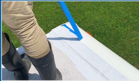
REMOVE PAINTER'S TAPE WHILE PRODUCT IS STILL WET TO PREVENT EDGE PULLING
