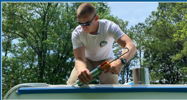
CAULK SEAMS WITH AN EVEN 1/4" - 3/8" BEAD
