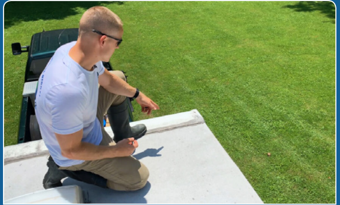
INSPECT PENETRATIONS TO SEE IF ANY AREAS NEED FIXING
