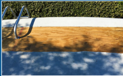
NEW WOOD INSTALLED
