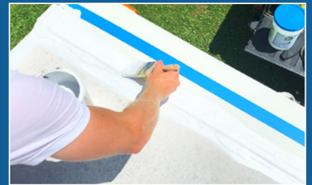
APPLY A LAYER OF CRAZY SEAL BASE LAYER OVER CRAZY PATCH
