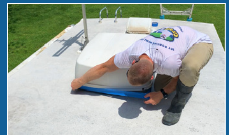
TAPE AROUND AC UNITS
