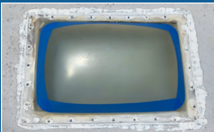
TAPE AROUND SKYLIGHTS
