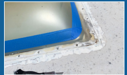
USE A KNIFE TO CUT ROUND CORNERS ON SKYLIGHTS
