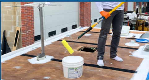
HAVE YOUR ROLLER FRAME READY WITH 1/2" NAP ROLLER ON AN EXTENSION POLE & CRAZY SEAL BASE LAYER
