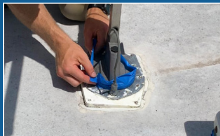
TAPE AROUND ANTENNAES
